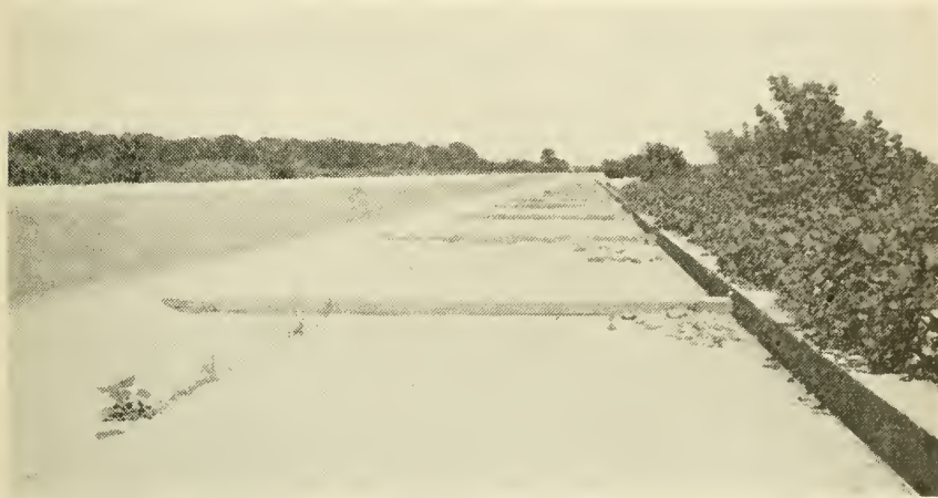
FIGURE 12. Fremont Weir. Top of weir is about eight inches lower at this point than elsewhere
