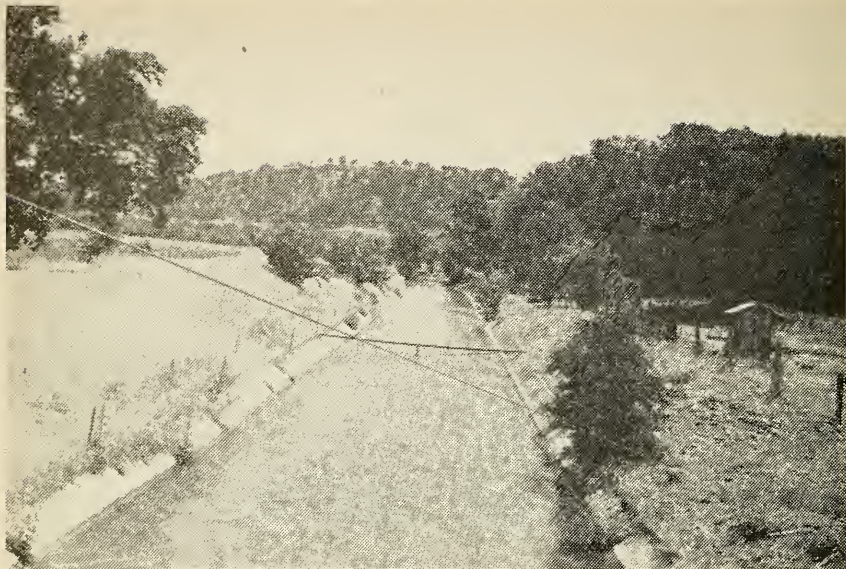
FIGURE 15. Diversion from south side of Capay Dam (Capay Canal), near take-off. June 18, 1940. Flow at time 303 second-feet
