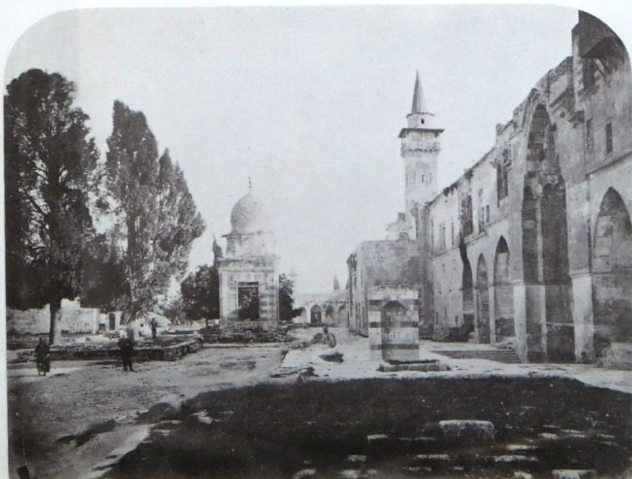
6b. WEST WALL AND CLOISTERS, LOOKING SOUTH
