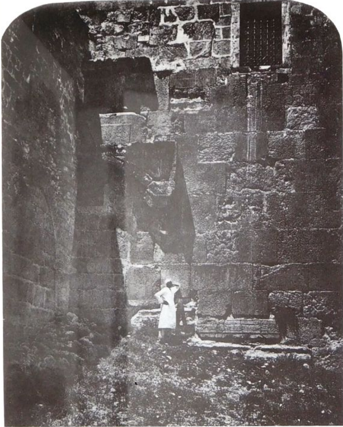
13a. DOUBLE GATEWAY IN SOUTH WALL
