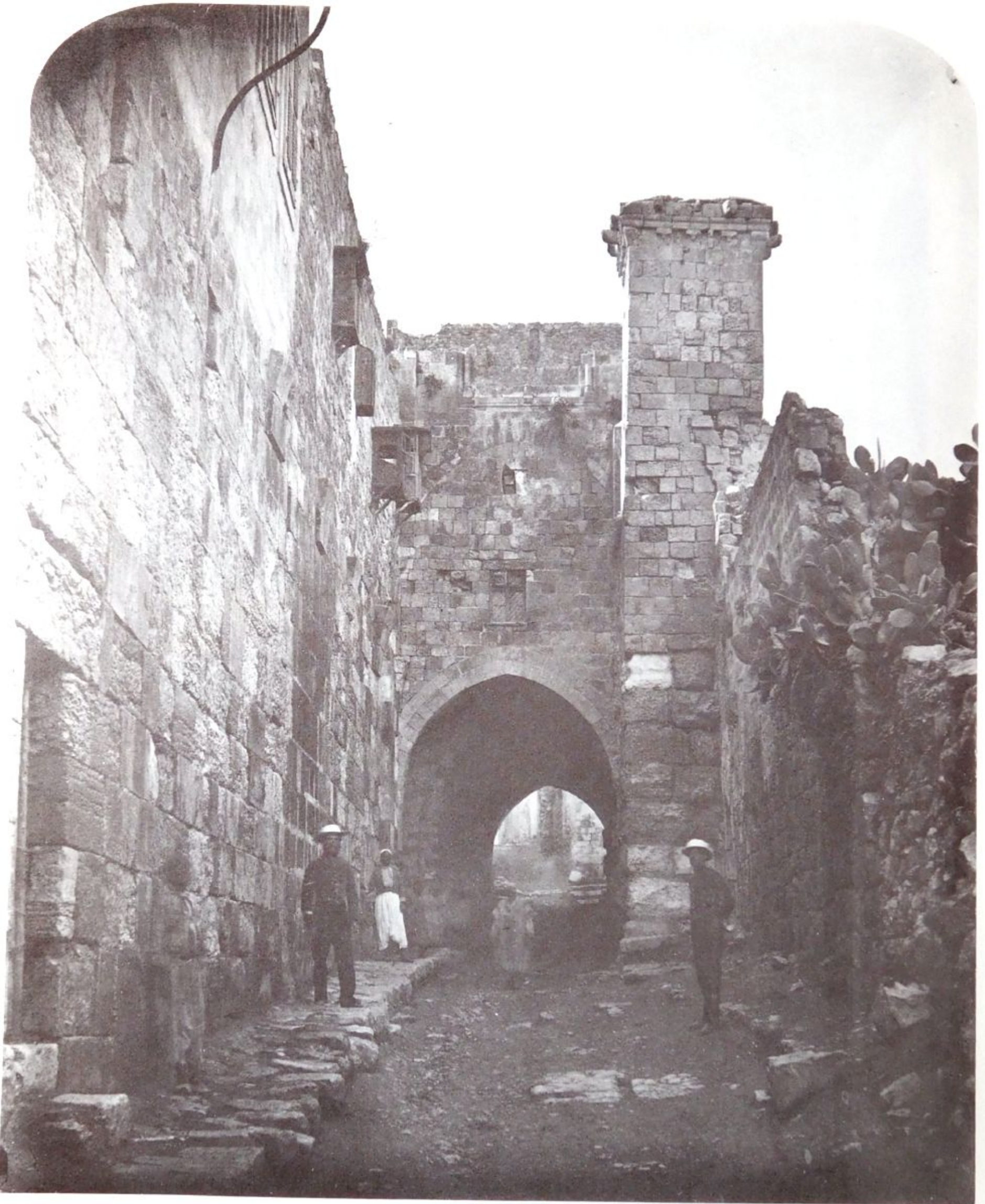
29a. THE SO-CALLED TOWER OF ANTONIA, IN THE STREET LEADING TO ST. STEPHEN GATE
