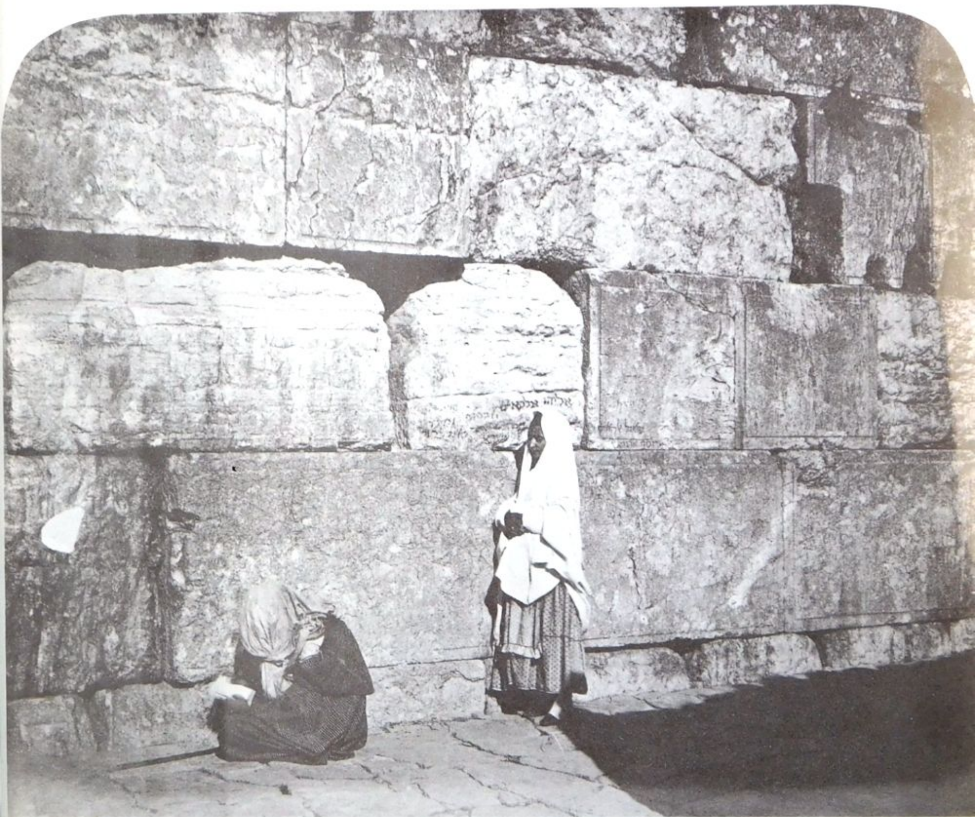
14b. DETAIL OF MASONRY AT WAILING PLACE
