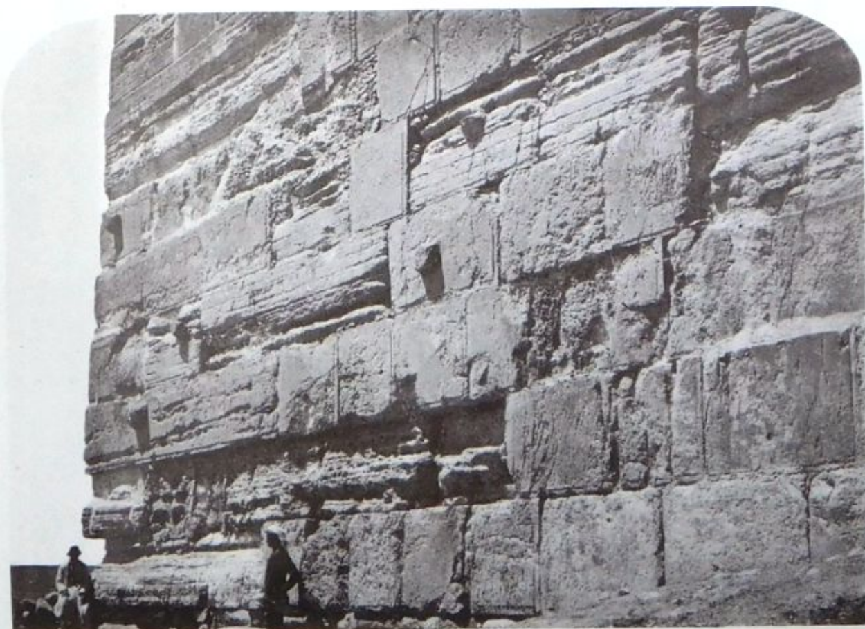
11b. EASTERN FACE OF SOUTH-EAST ANGLE
