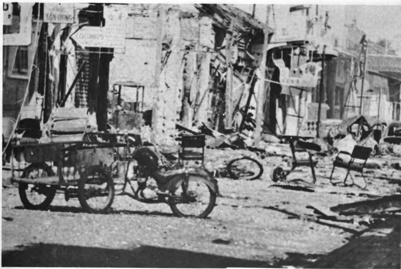
A barricade erected with furniture and vehicles on Nguyen Trai -
