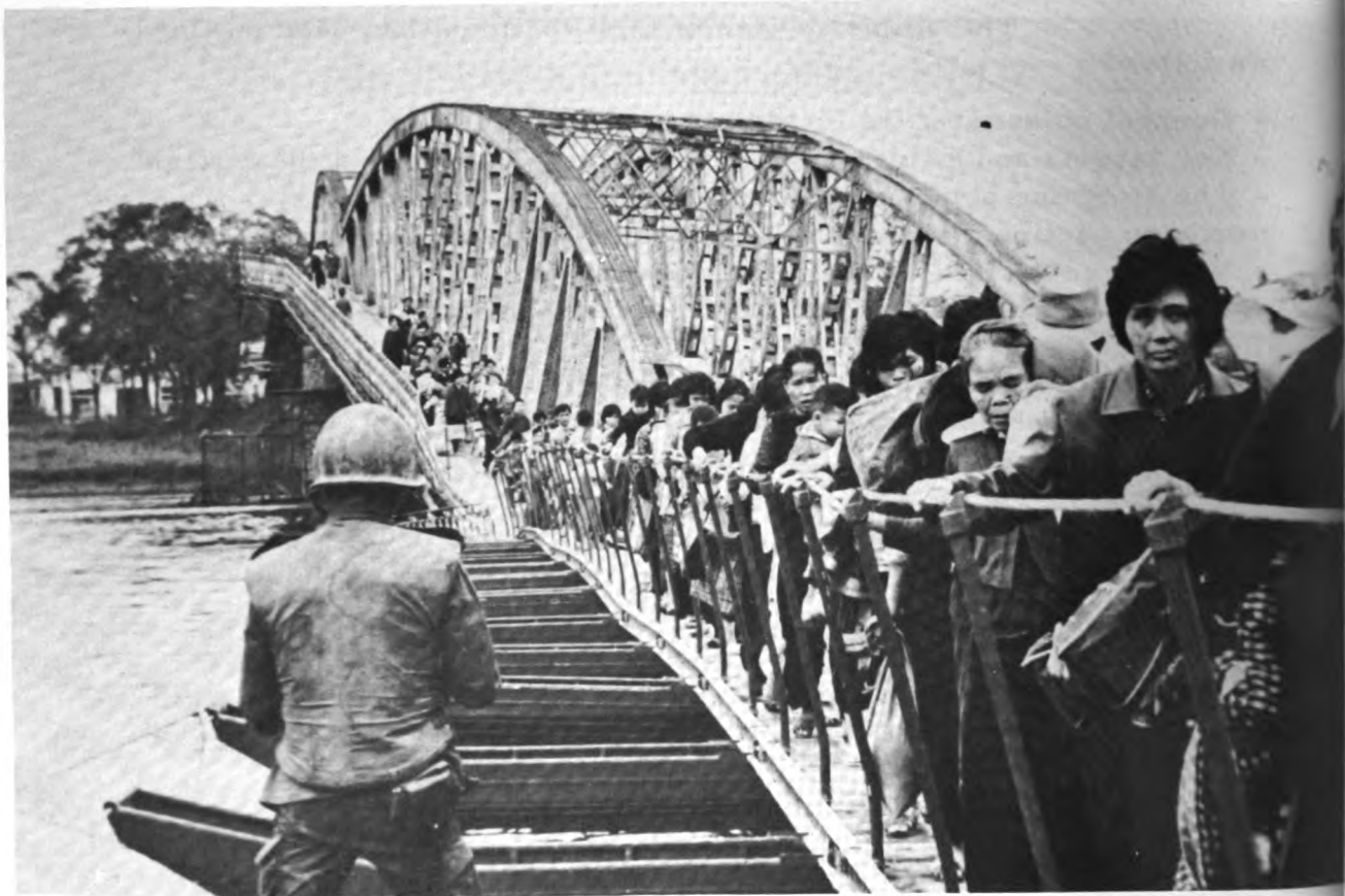
After the arrival of engineer troops, two narrow lanes were immediately launched for the people's use.
