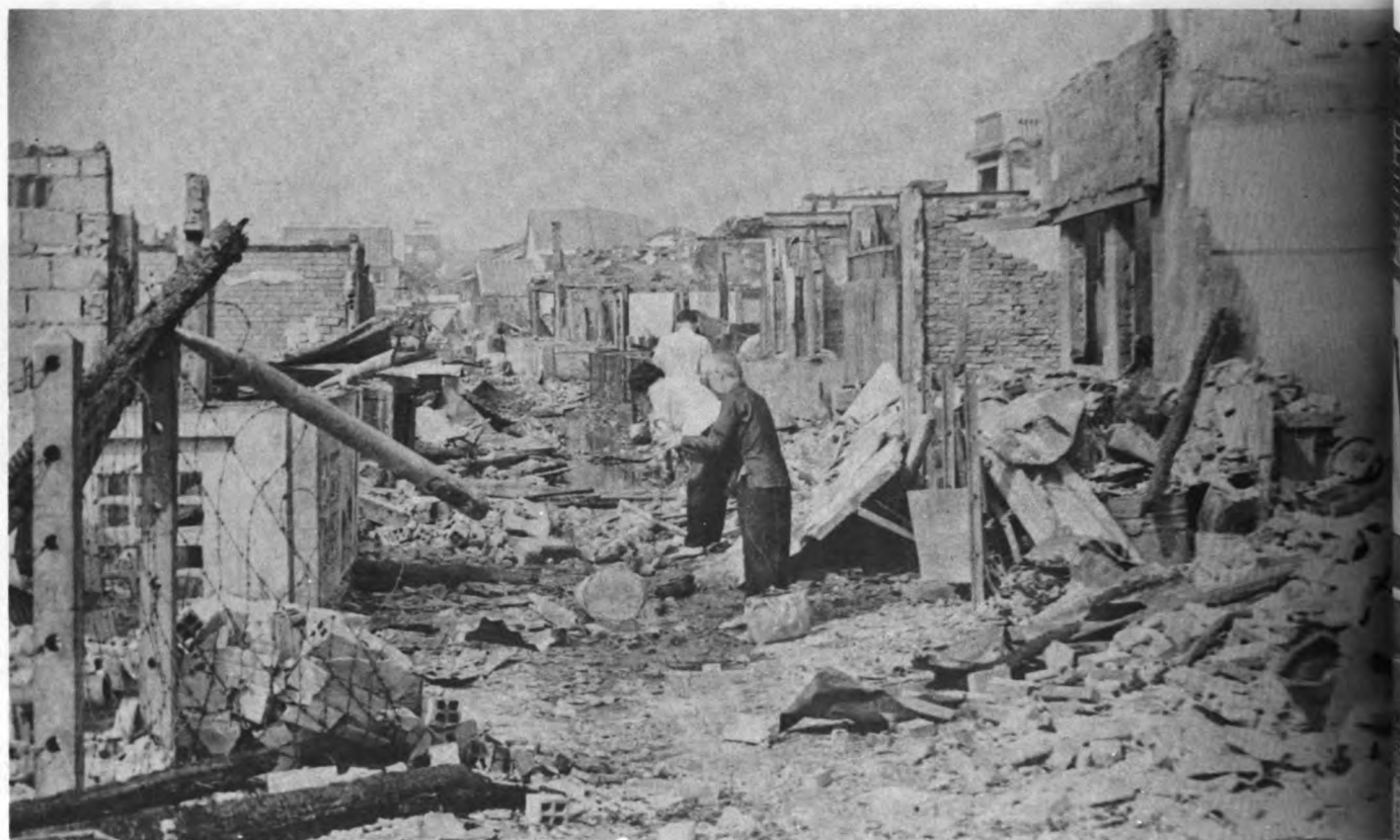
The Ban Co area after the big fire of 7 February 1968.
