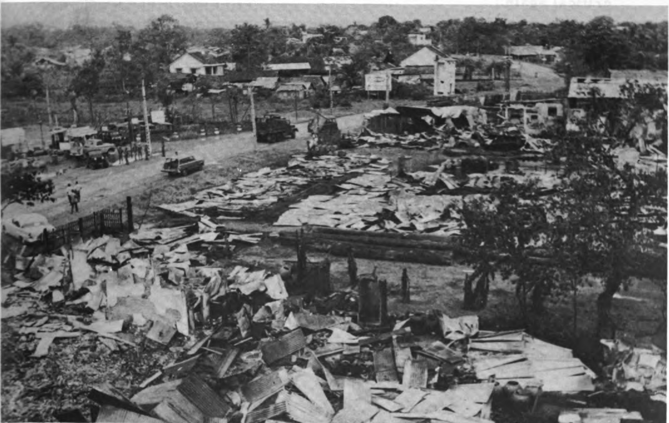
Scene of area in vicinity of Bang Ky Bridge. Thuan Loi timber plant in ruins
