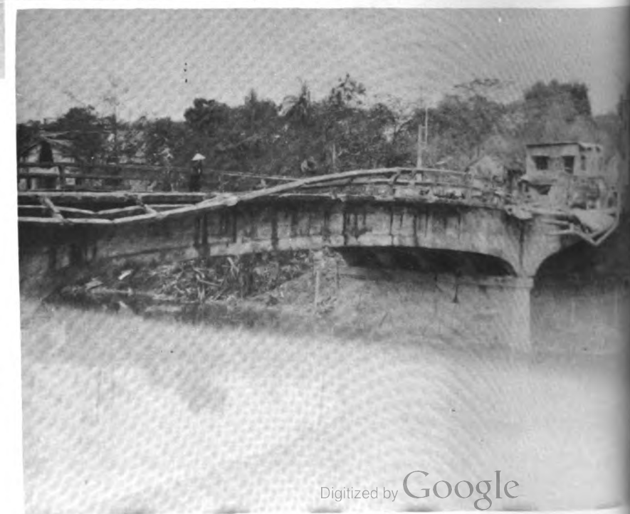
The Ben Ngu Bridge was only slightly damaged.
