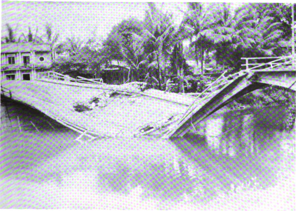
The Phu Cam bridge. It was to be rebuilt.
