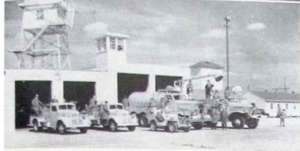
Top: Gas station, 578th AMS Above: Line Fire Department, 35AES
