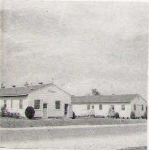
Communication and Public Relation Office Building
