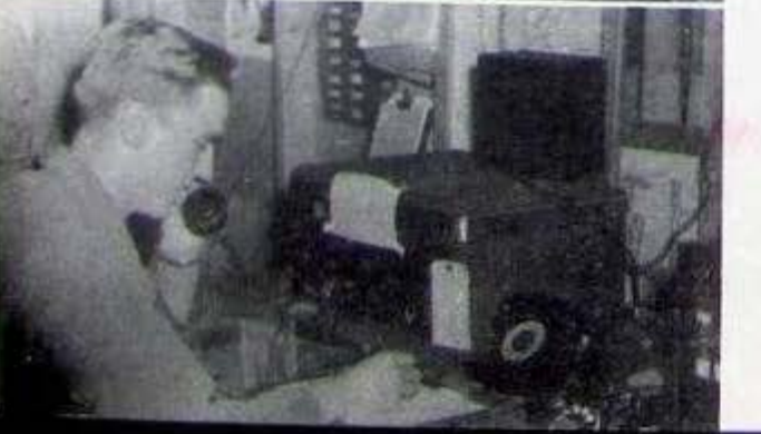
Alarm and crash fire station
