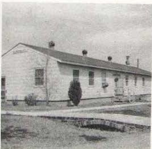
Station Signal Office
