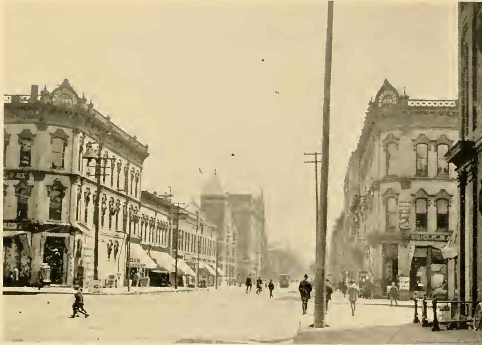
THIRD STREET, LOOKING SOUTH FROM FIRST AVENUE
