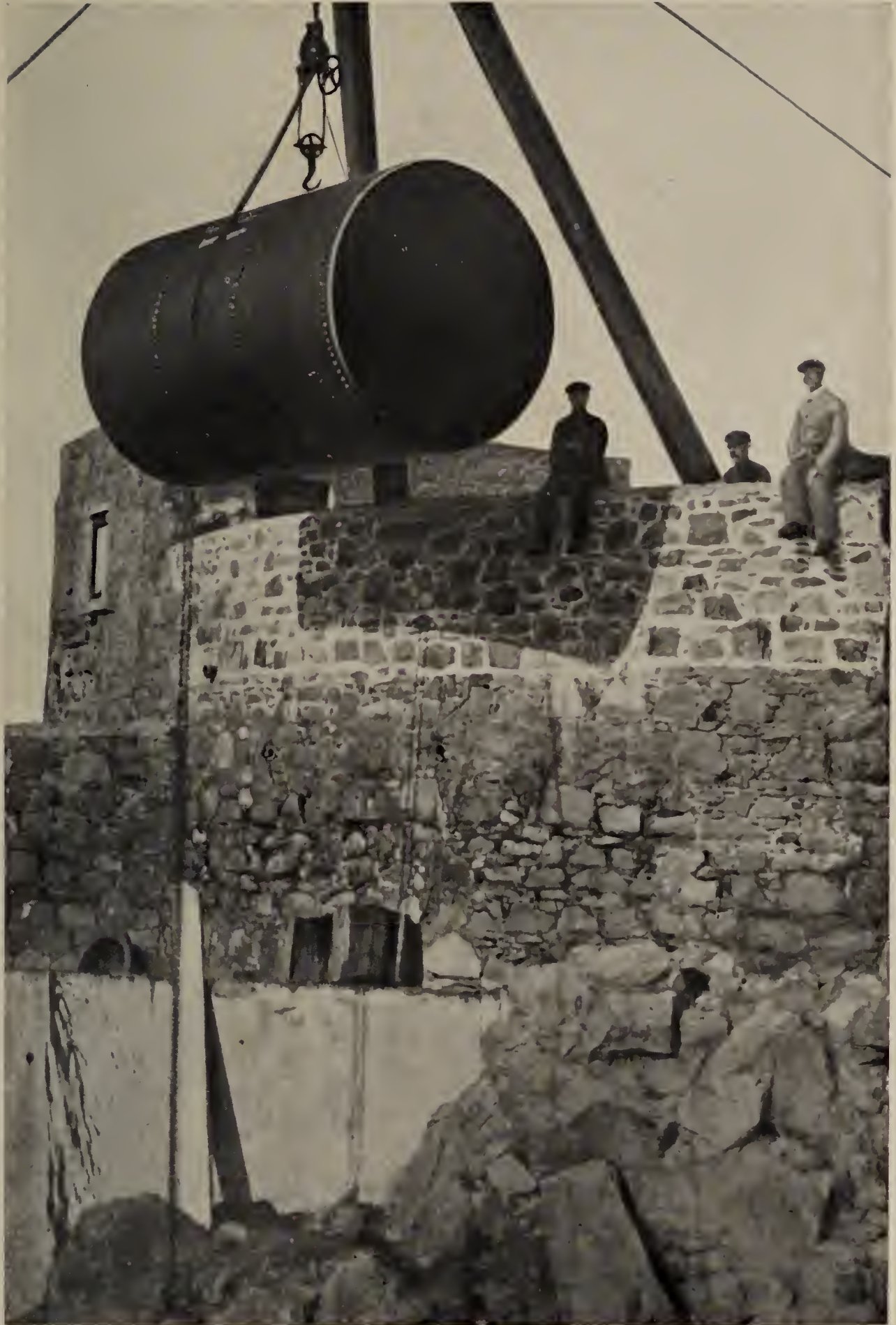
SETTING THE COMPRESSED-AIR RESERVOIR AT FORT DOYLE.
