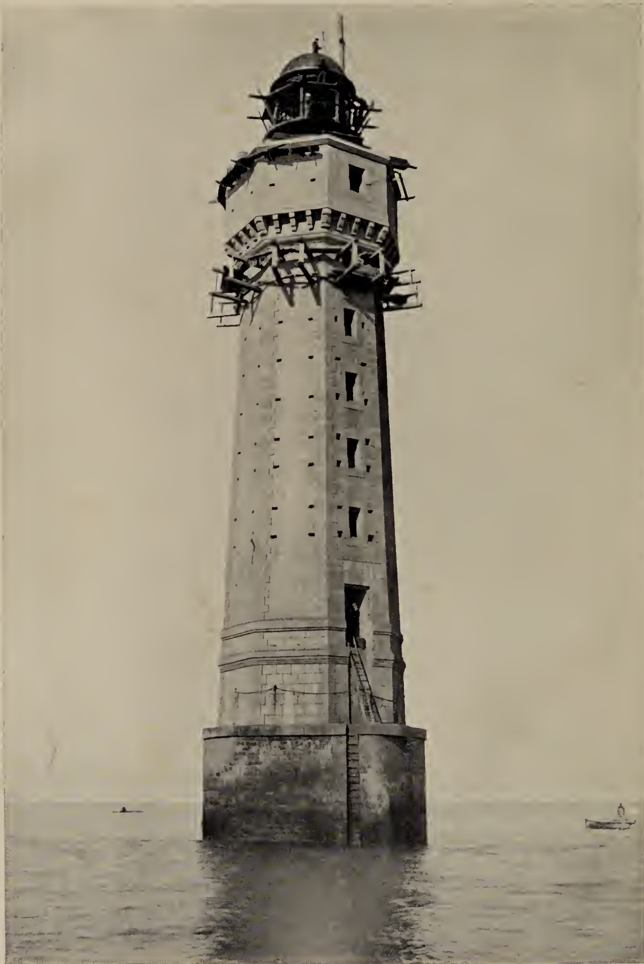
FITTING THE LANTERN OF LA JUMENT LIGHT.
