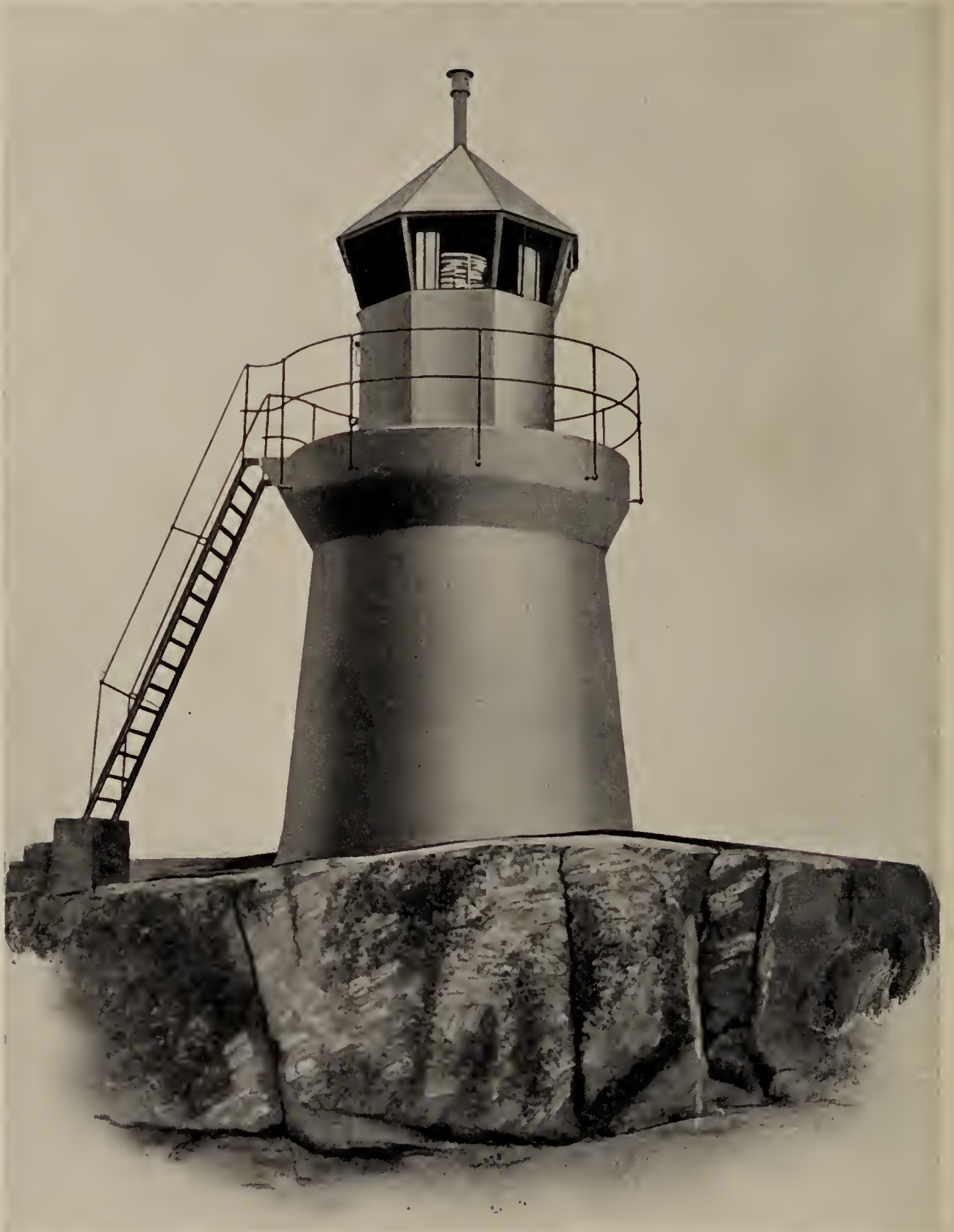
THE GASFETEN LIGHT : A LONELY BEACON IN SWEDISH WATERS.
