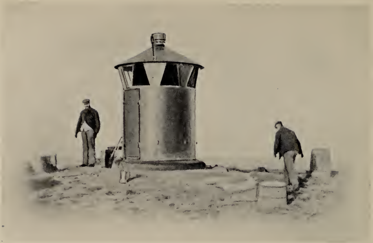
AN UNATTENDED BEACON LIGHTING THE STRAITS OF MAGELLAN. This warning, fitted with Dalén flasher and sun-valve, is visited once in six months.
