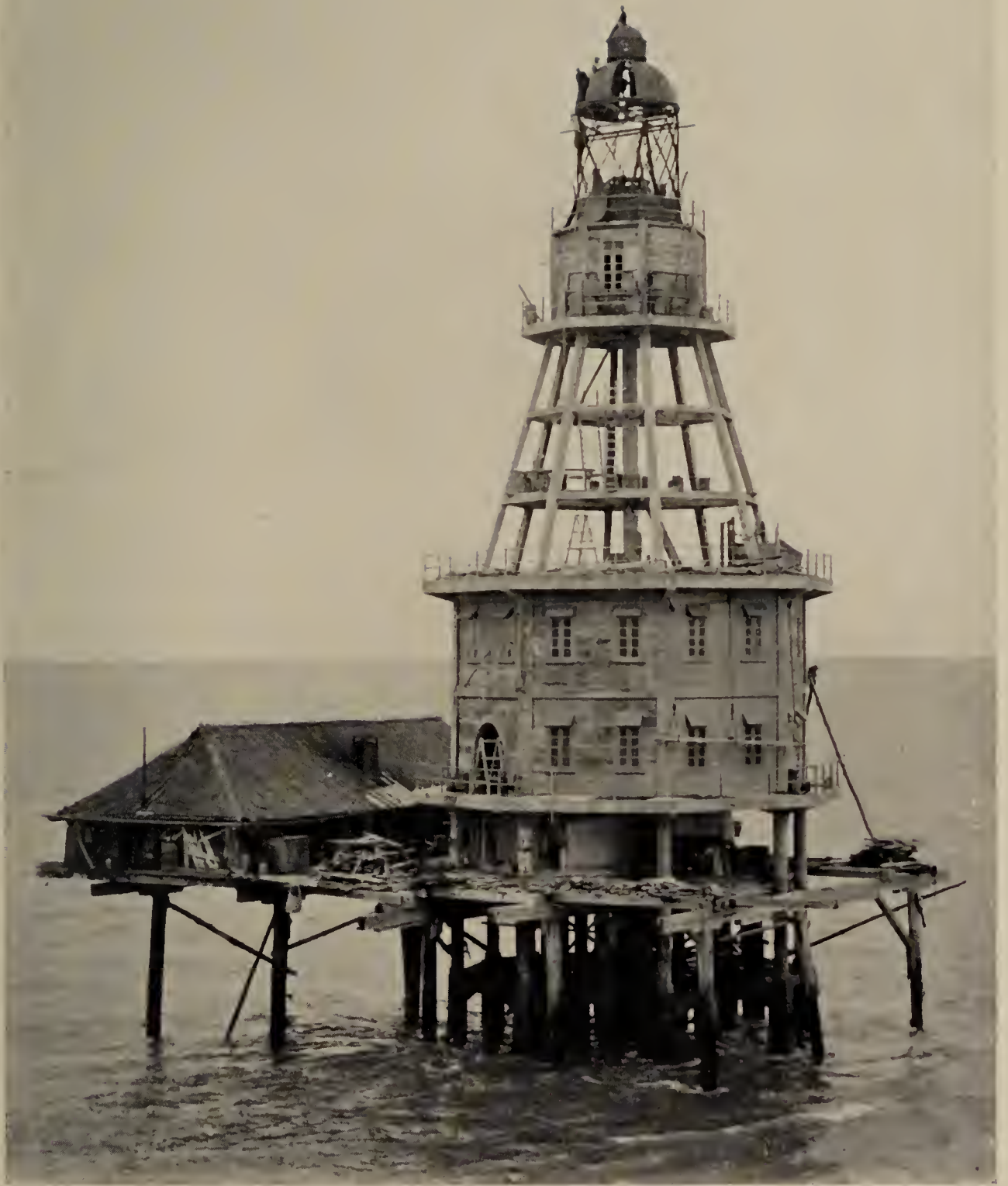
COMPLETING THE ONE FATHOM BANK LIGHTHOUSE IN THE MALACCA STRAITS.
