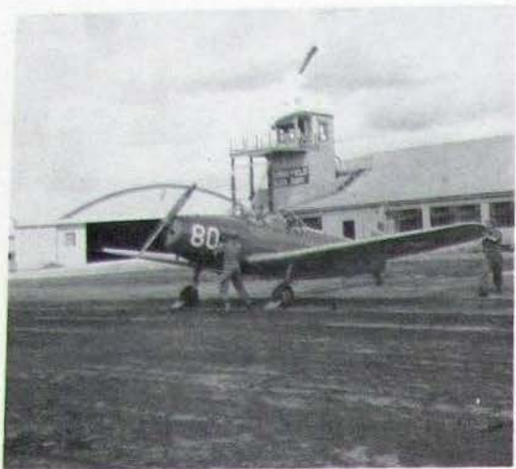
The control tower.
